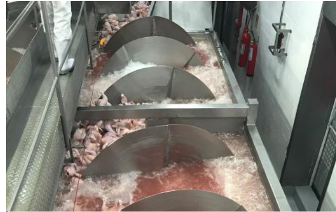
The majority of refrigeration should be added in the final third of the chiller
