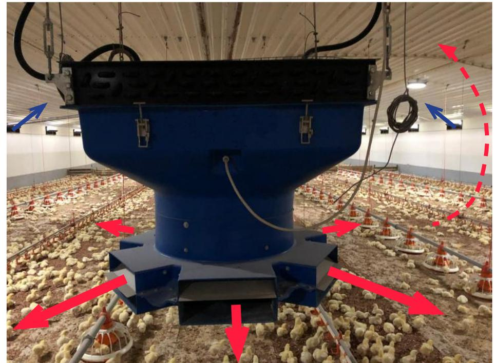
An illustration of a vertical circulation fan system. The thick red arrows show high velocity distribution and a thinner dashed red line shows the return air going back to the ceiling. The thick blue arrows indicate the cold air coming in through the perimeter inlets.
