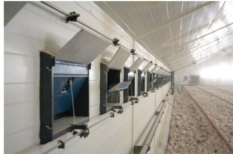
*In non-tunnel ventilated houses the high pressure fogging nozzles are installed along the perimeter wall just above the perimeter inlets. The number and capacity of the nozzles, will depend on the target temperature drop created through evaporative cooling*
