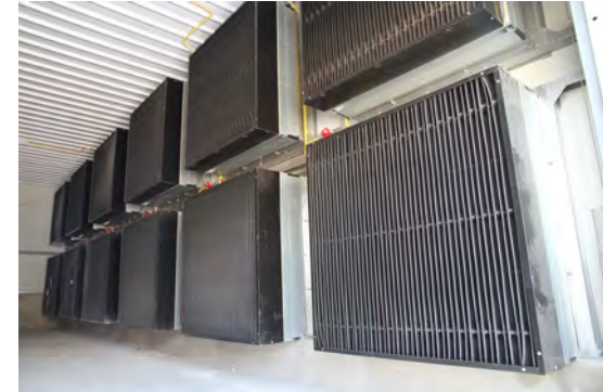
Light traps mounted over fans can reduce fan performance, and are not the best option in a high-speed tunnel houses.
