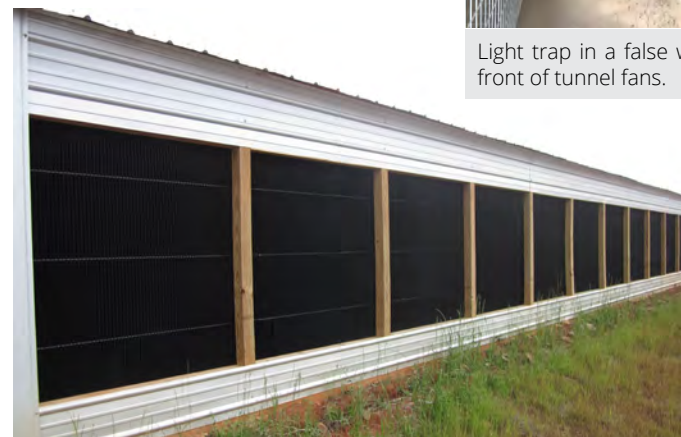
Tunnel inlet light trap.
