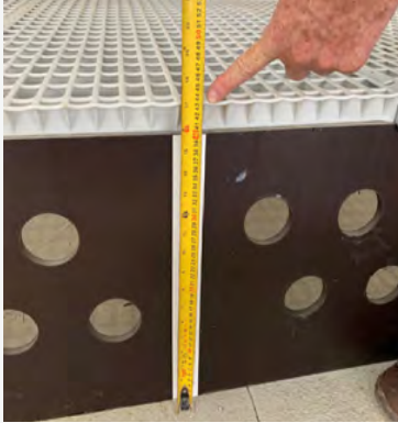
Slats should be 45 cm (18 in) high, measured from the top of the slats to the concrete floor.
