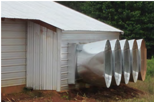
Tunnel fan light trap false wall installed in “dog house” or plenum in front of tunnel fans installed on the sides of the house.
